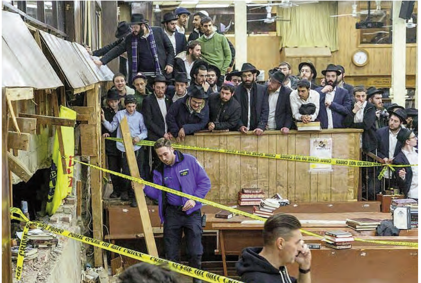
Hasidic Jews tunnel beneath Jewish synagogue in Brooklyn.
